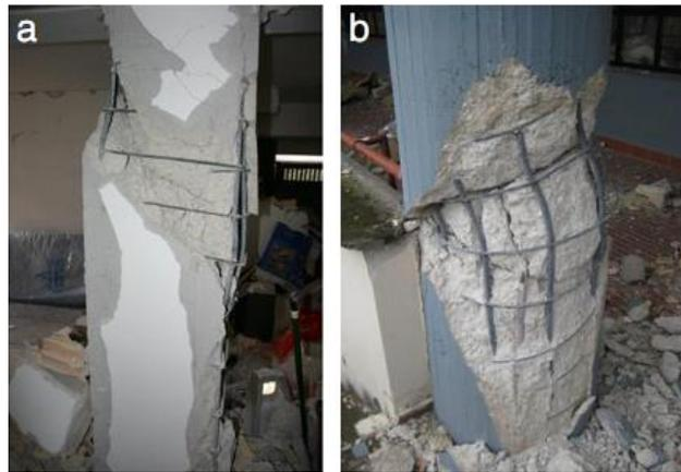
Figure 1 : Shear Column and Circular Column situation in Earthquake
